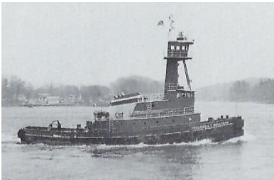
The Fredrick E. Bouchard , shown above, was built in 1975 for Bouichard Transportation by Halter Marine, New Orleans. She measures 104.6' x 31.1' x 16.4' and powered by 3900-horsepower diesel engine. Though smaller than the Intrepid she performs most of the same tasks.
